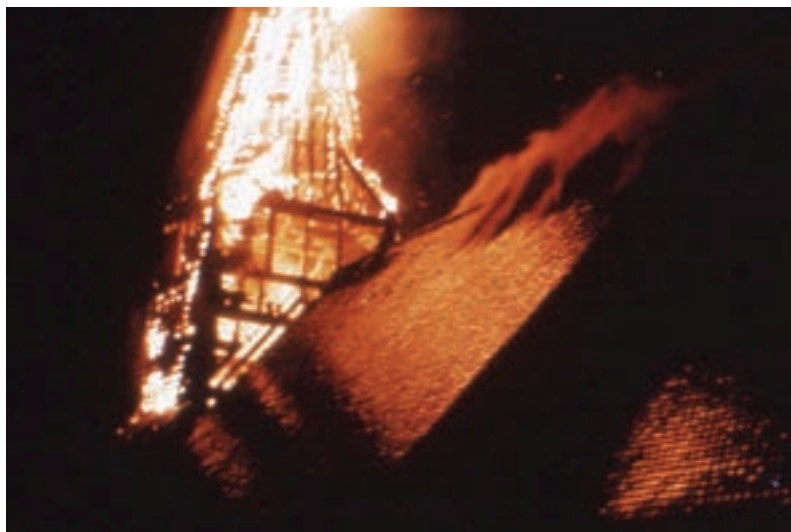
Fire following a lightning strike on the eve of the Fair 1964
